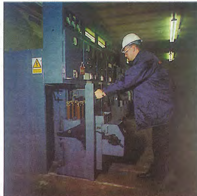
Project Engineer Dave Parry testing and commissioning the HV switchgear.
